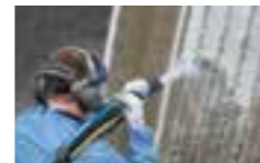
8.6 to 10 bar: Abrasive blasting
