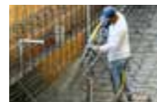
7 to 12 bar: Shotcrete applications
