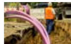
12 to 14 bar: Cable blowing and drilling
